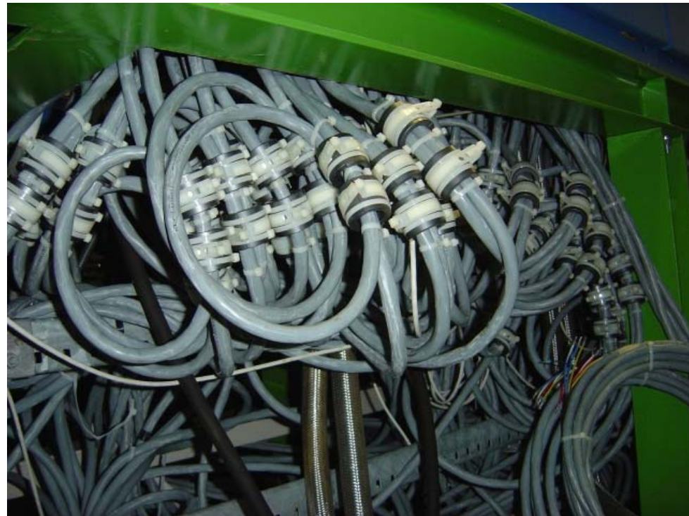
24 x TESLA 3ch 200V PS in USA15. Mounted ferrites on 200V cables.
