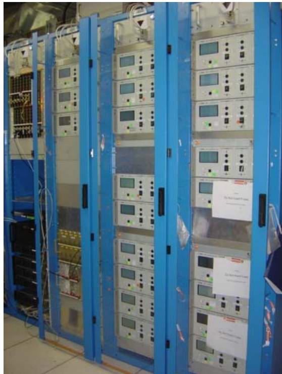
24 x TESLA 3ch 200V PS in USA15. Mounted ferrites on 200V cables.
